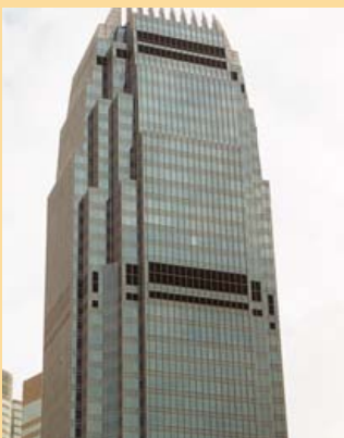
Fire refuge floor
