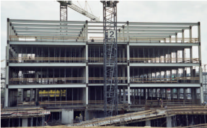
Figure 2. Side view of the building during construction
