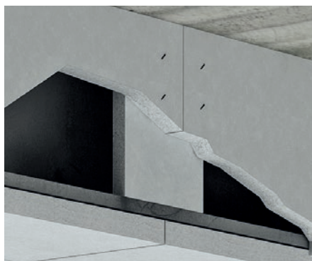
Butt joint detail of fire-protection cladding
