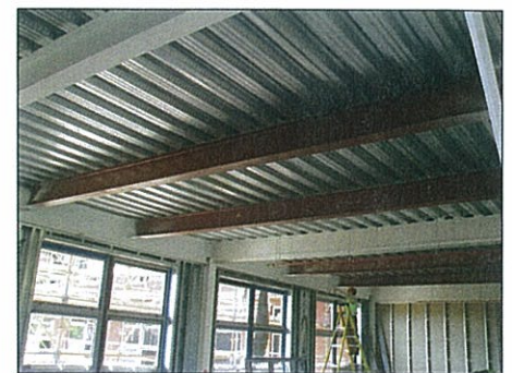
Fig. 13: Project showing unprotected beams and protected beams utilising latest design methods incorporating membrane action
