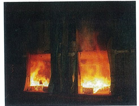
Fig. 16: Fire test on a seven-storey concrete-framed building
