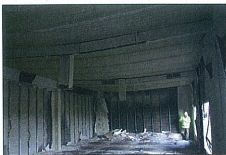
Fig. 5: Picture taken after a full-scale fire test showing the loss of protection to the steel beams which occurred at the height of the fire
