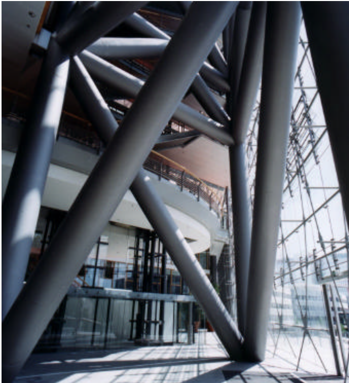
Figure 4. Truss tower made of hollow sections (Copyright by ThyssenKrupp Stahl AG)
